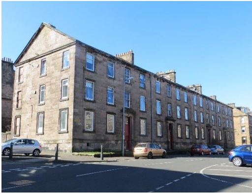
Figure 25 Windows replaced in uPVC
