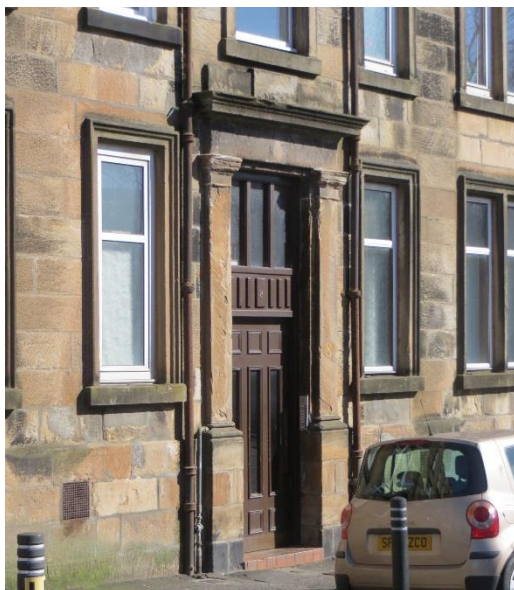
Figure 24 Cement-based repairs
